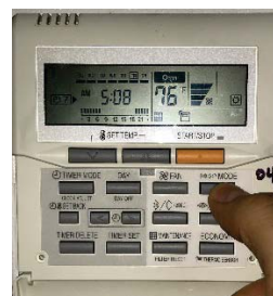
Ex.2- The role of the remaining RC's will be selected automatically.
